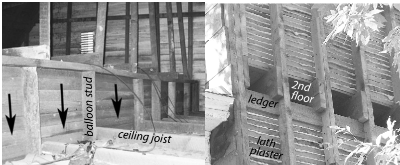
Balloon framed walls: Wall cavities, shown from outdoors at right and from the attic at left, are open to the floor cavity, the attic, and the crawl space.
