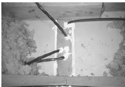
Leaky top plates: The cracks along top plates are from lumber shrinkage. They are small cracks but there are long lengths of them.
