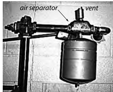
Expansion tank, air separator, and Vent: Preventing excessive pressure and eliminating air from the systems are important for hydronic distribution systems.
