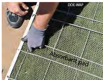
Cooler pads: Pads collect dirt and scale. Replace them when cleaning is ineffective.
